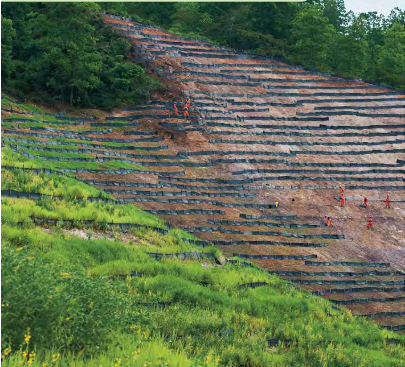
Concurrent rehabilitation of a waste rock dump at the Pueblo Viejo mine in the Dominican Republic.
