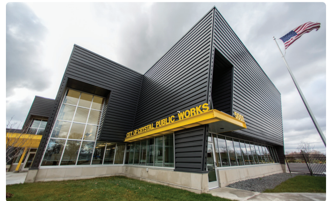
CITY OF CRYSTAL PUBLIC WORKS | Crystal, MN Big-D Construction’s public facility experience spans the country. Above is recently completed project by Big-D Midwest in Minnesota.
