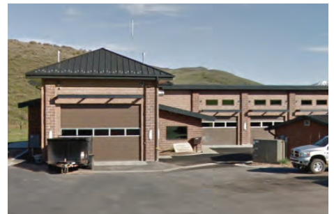
Summitt Water Distribution Company Office & Operations Building
