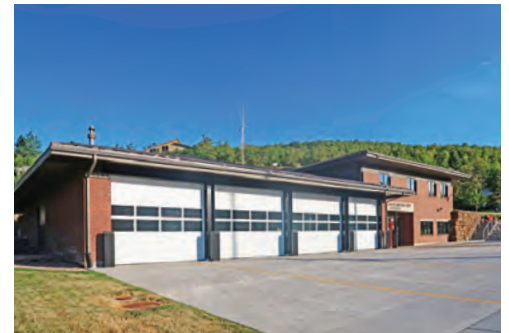
Mueller Park #84 Fire Station Seismic Upgrades & Remodel
