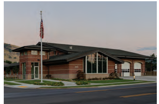
Centerville Station #83 Fire Station Replacement
