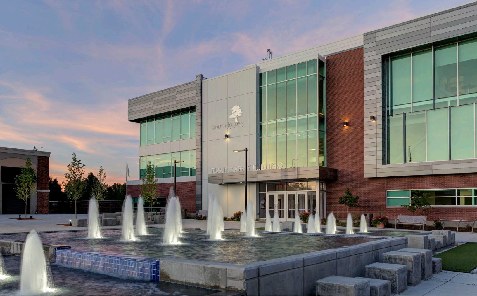
South Jordan Public Safety Building
