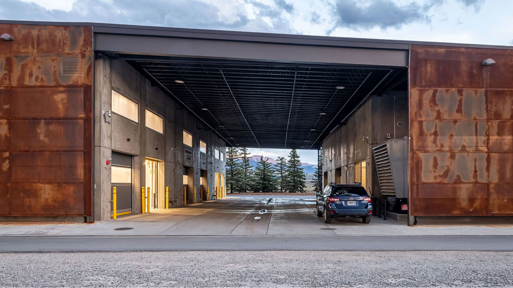
Jackson Airport Landslide Project
