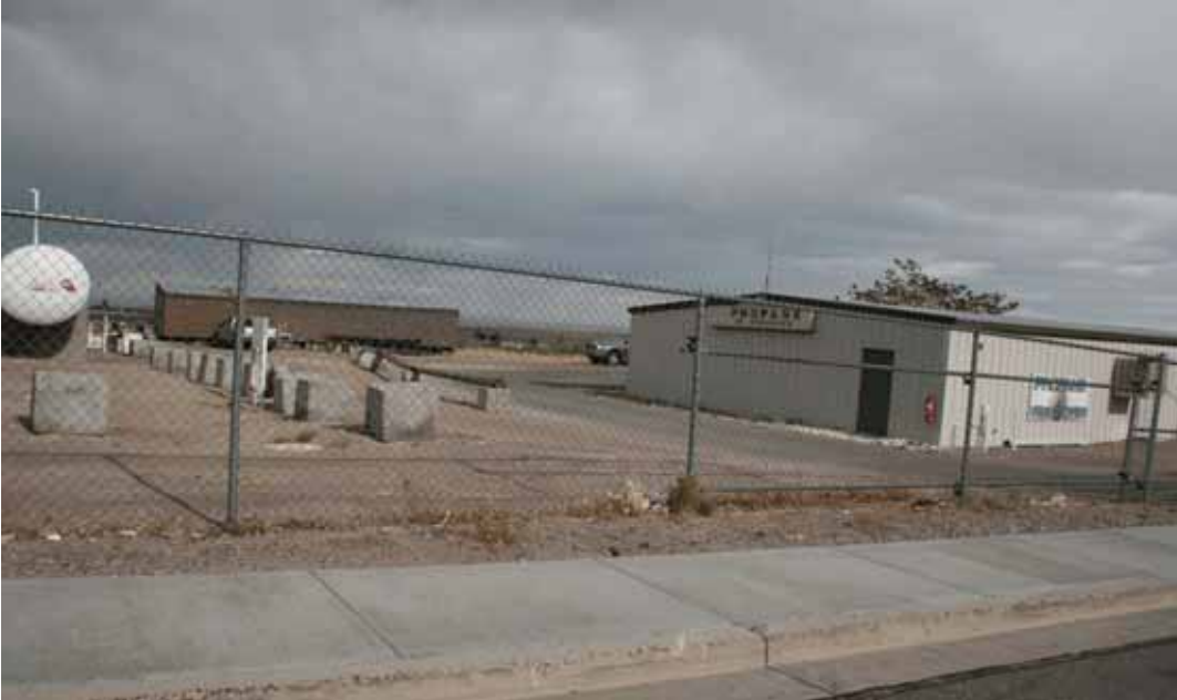
General view of a mid-portion of the subject improved property looking southeasterly from near its westerly mid-limits and Mesa Street
